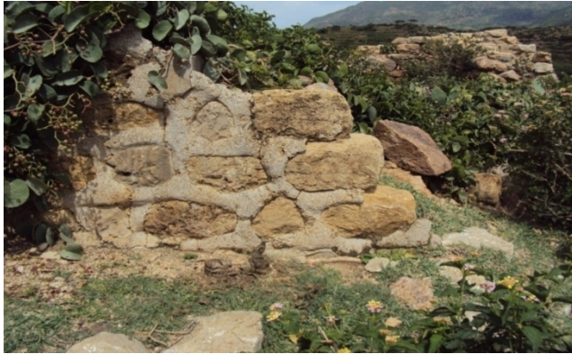
Source: Photo taken during observation/field research: 2008 (E.C)
